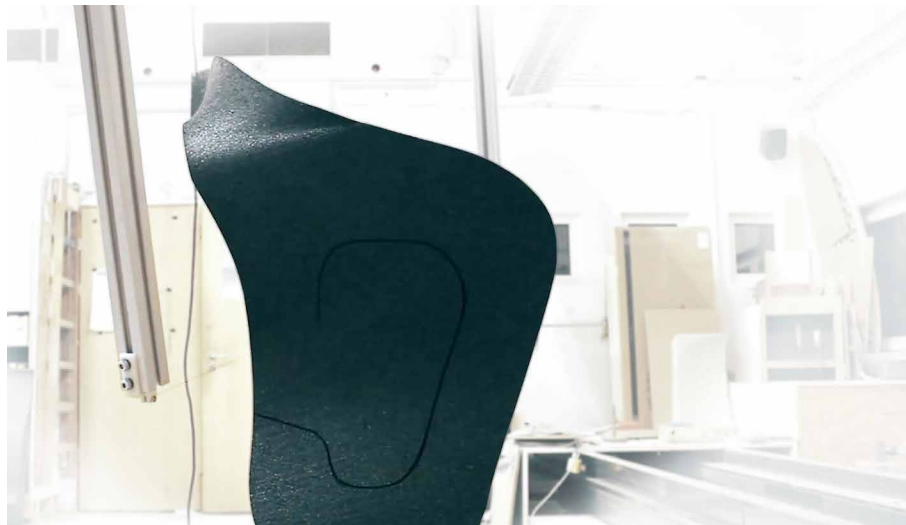
FIG. 4.28 Robotic Hot Wire Cutting of the developed surfaces of the Hybrid Chair.
