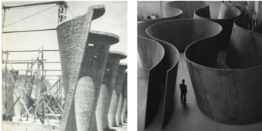
FIG. 2.18 Left: Undulating Cantilevered Brick Wall in Estación Atlántida, 1960, Uruguay, Eladio Dieste; Right: NJ-2, Rounds: Equal Weight, Unequal Measure, Rotate by artist Richard Serra; The curvature of the wall and variation in the horizontal section result in stability of the building and the large-scale sculpture.
