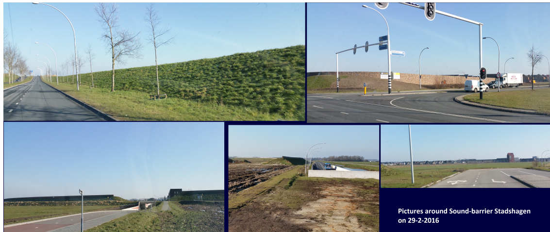
Figure E.2: Impression of the sound-barrier in February 2016. Locations that were finished in the top, the picture in the bottom left a tunnel that has to be closed in case of a flood, location where the sound barrier abruptly stops because neighbourhoods are not yet developed as can also be seen with the end of a road in the bottom right of the figure.
