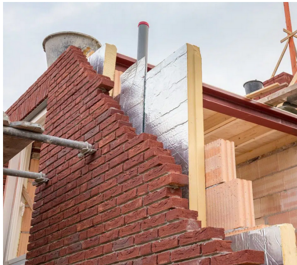
Figure 3.1: Cavity wall [64]
