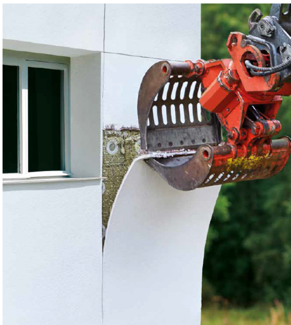
Figure 5.3: Weber.therm circle demolition practice [63]
