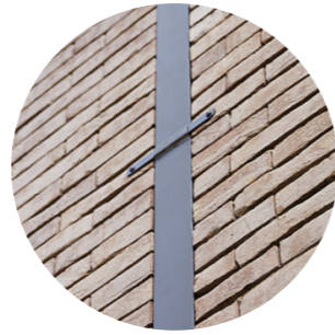
Aluminium rainwater pipe
