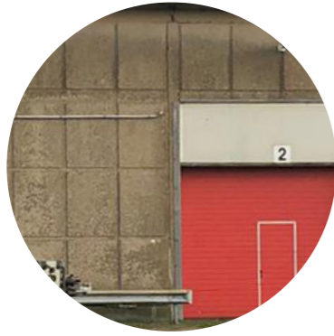
Brick with vertical (concrete) lines aligned with wooden window frame
