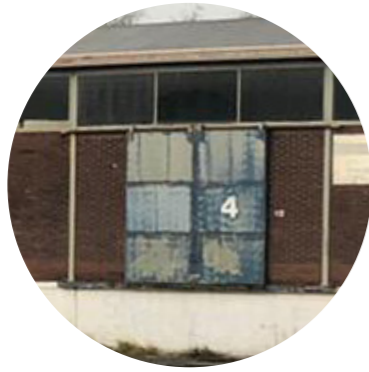
Brick with vertical (concrete) column aligned with wooden window frame
