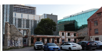
Rotermann district ruin - parking and two industrial halls
