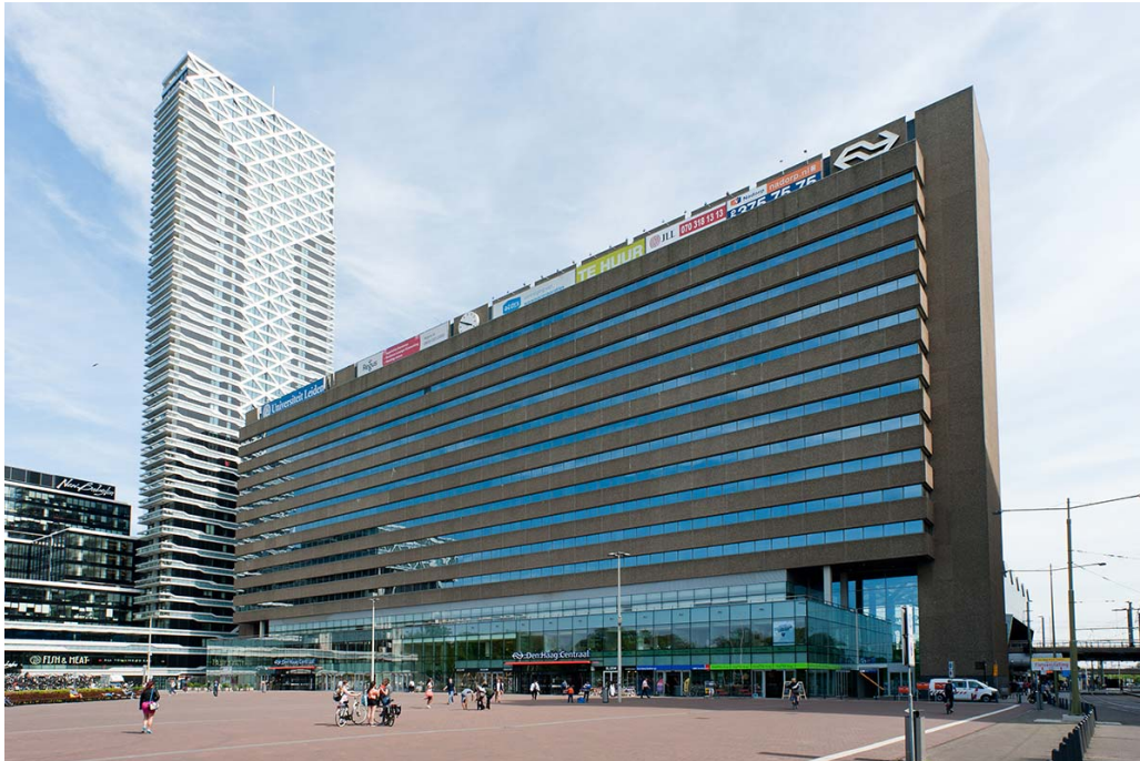
Figure 6.2: Stichthage Building (Diagonal View)
