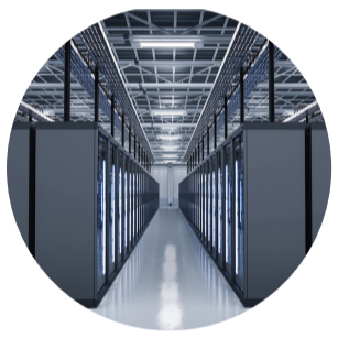
Data Centre Heat Re-use
