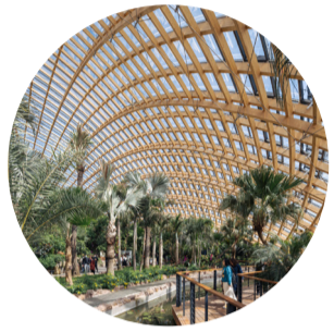
Lightweight Glulam Timber Skeleton + Gridshell Roof
