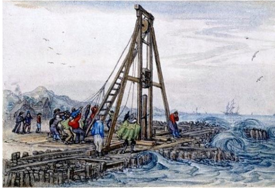
Figure 2, Left - Wooden palisades in the water were applied with manpower. [8] Figure 3, Right - Amsterdam foundation [7]
