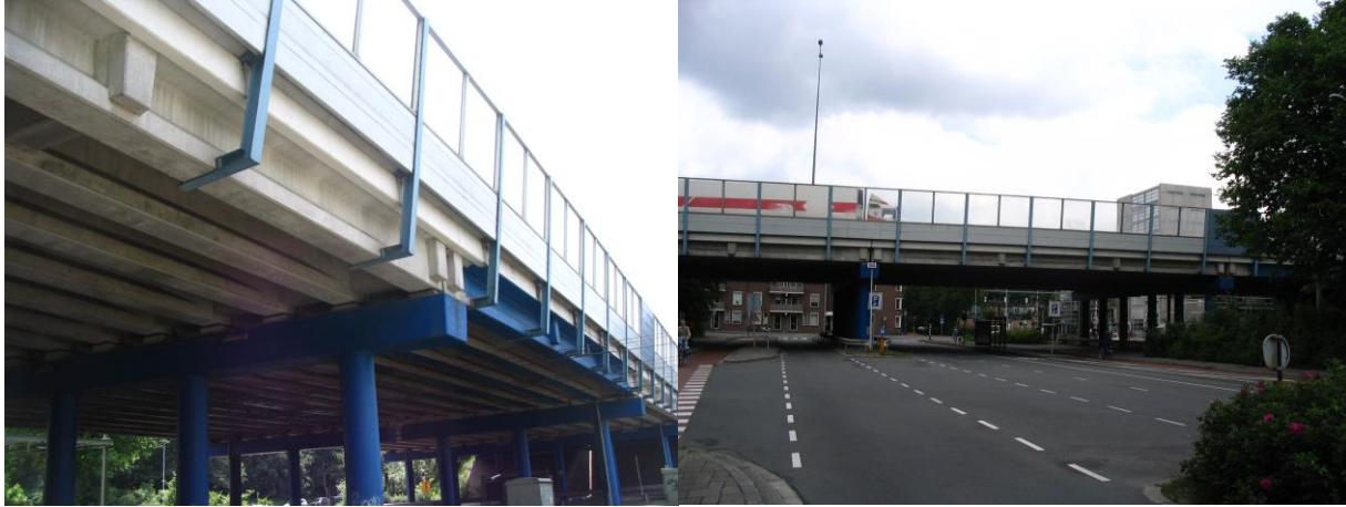
Figure 1.9 Bridge Deck in Helperzoom, Groningen, Netherlands
