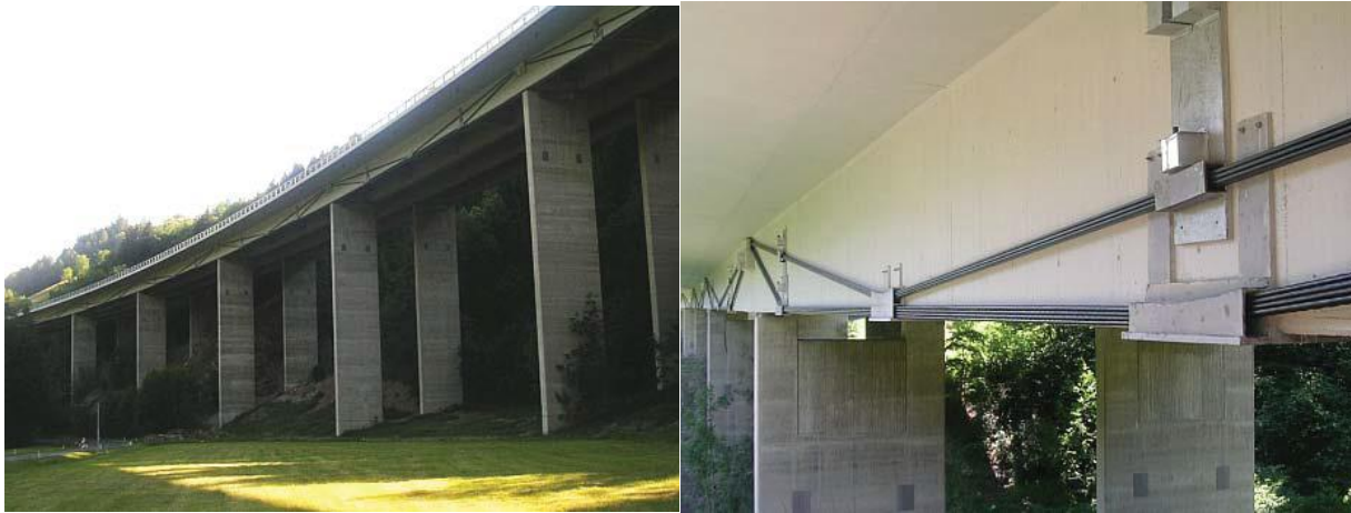
Figure 2.2 Strengthening by external post-tensioning in bridge decks [20]
