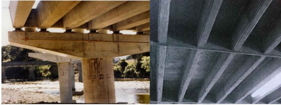
Figure 1.7 RC beams supporting bridge decks and slabs [15] [16]
