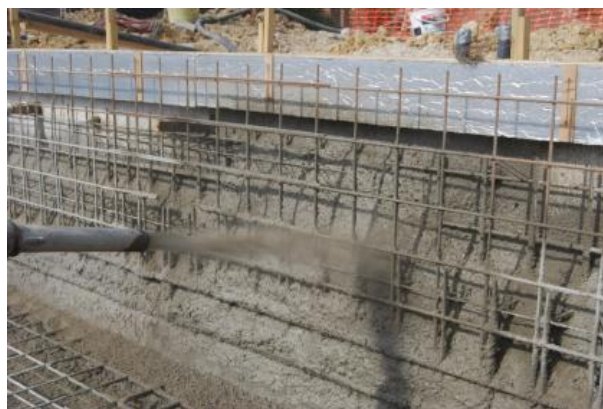
Figure 2.3 Strengthening by reinforced shotcrete [18].
