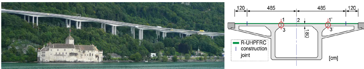
Figure 3.5 Chillon viaducts along Lake Geneva and the geometry of the box girders cross-section [38].
