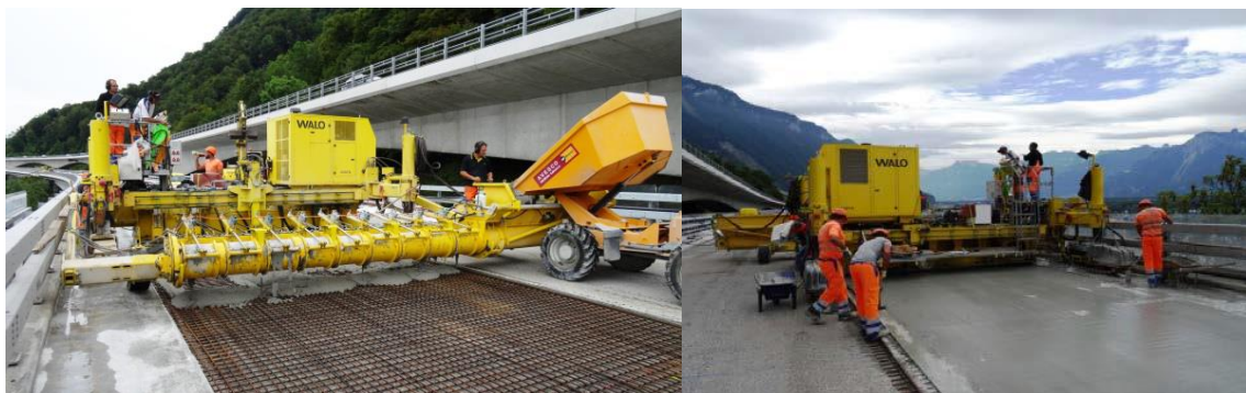
Figure 3.6 Application of R-UHPFRC on the decks of Chillon Viaduct [28]
