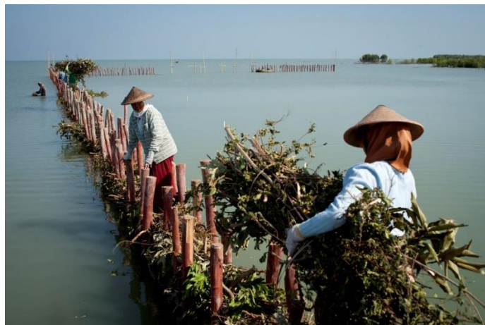
Figure 59 Construction of a permeable dam
