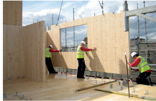
■ CLT walls and floors are prefabricated and therefore construction time is drastically decreased comparing to traditional building (image: Simpson Strong-Tie)
