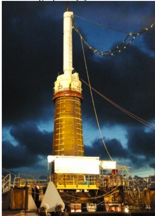
Figure 2: Impact driving with a hydraulic hammer at the Riffgat project [4]
