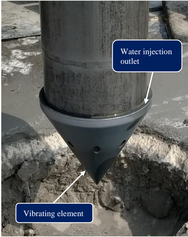
Figure 10: Vibrating element attached to the foundation pile.
