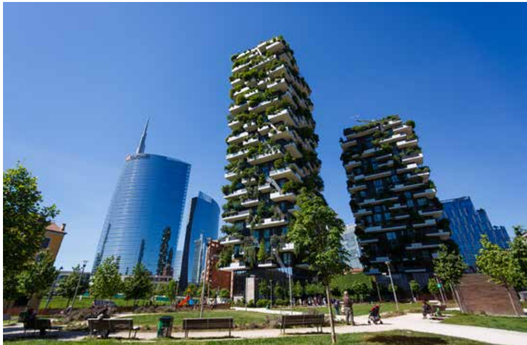
FIG. 3 Bosco Verticale with the UniCredit Tower behind in Milan, Italy. (Source: Konstantin Tronin / Shutterstock.com)
