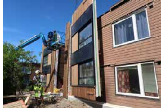
FIG. 6 4RinEU facade installation sample, external side view (source: Municipality of Oslo)
