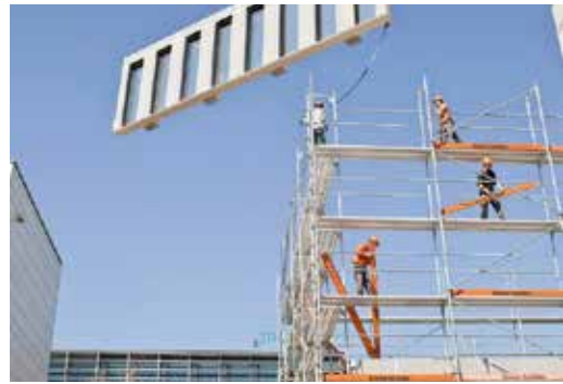
FIG. 10 Installation of LCT ONE facade system through scaffolds (source: ww.creebyrhomburg.com ©Darko-Todorovic|Photography|adrok.net)
