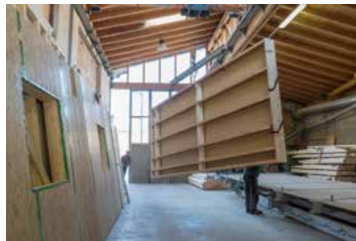
FIG. 8 SINFONIA project – panel production (source: Benedikter Architekten)
