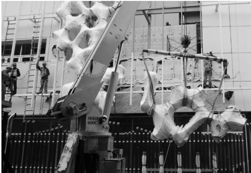
FIG. 12 Module segments during installation, bolted to painted metal sub-framing (Elegant Embellishments, 2018)
