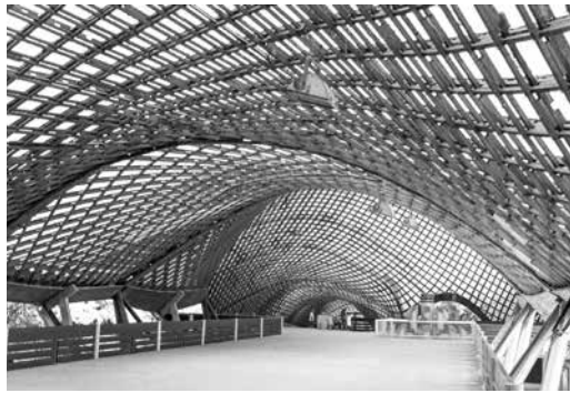
FIG. 1 The Multihalle in Mannheim, Germany (Carlfried Mutschler with Frei Otto)
