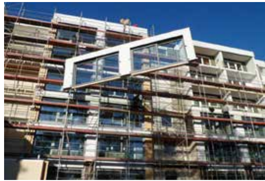
FIG. 2 TES EnergyFacade project – panel installation (source: Gumpp & Maier)
