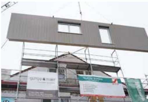
FIG. 3 iNSPiRe facade installation sample, external side view (source: Gumpp & Maier)
