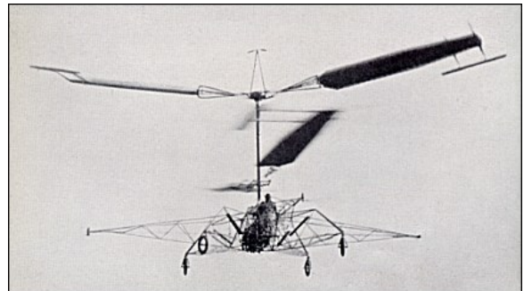
FIGURE 1. CORRADINO D’ASCANIO’S HELICOPTER WITH SERVO TABS.
