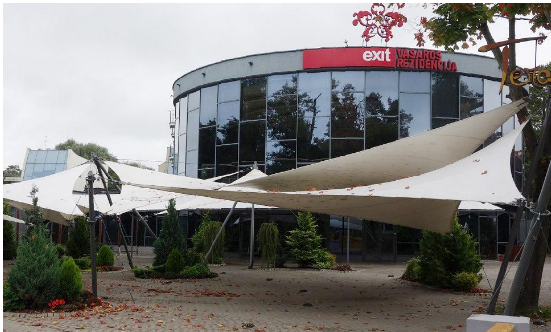
Figure 18: The appearance of the facade after reconstruction at the daytime, 2016.
