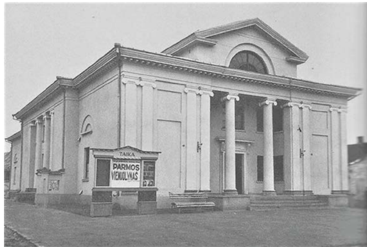
Figure 1: Stalinist period cinema building “Taika” transl. “Peace” in Kaunas. Built in 1953, standardised project.
