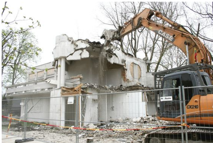
Figure 11: Demolition of cafe “Banga” in 2015.
