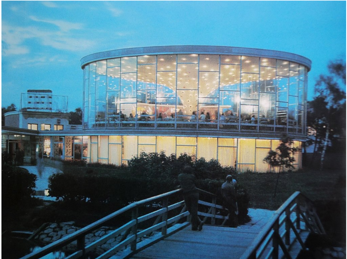
Figure 19: Original design of the restaurant "Vasara" by night. Arch. A.Eigirdas. Built in 1964. Photo: 1973.
