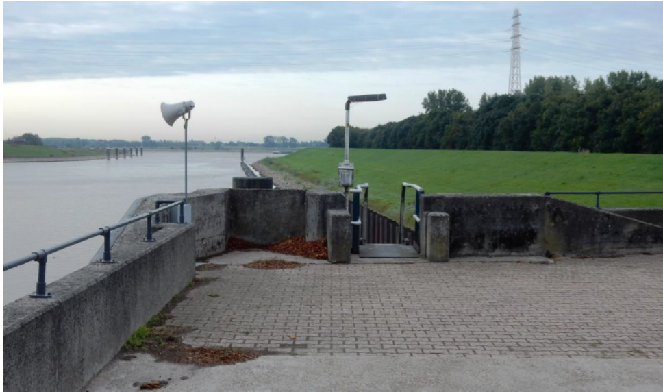
Figure 6.4: Retrieving wall at the Prins Bernard lock. The openings in the wall are closed off during extreme conditions. Retrieved from Rijkswaterstaat (2019).
