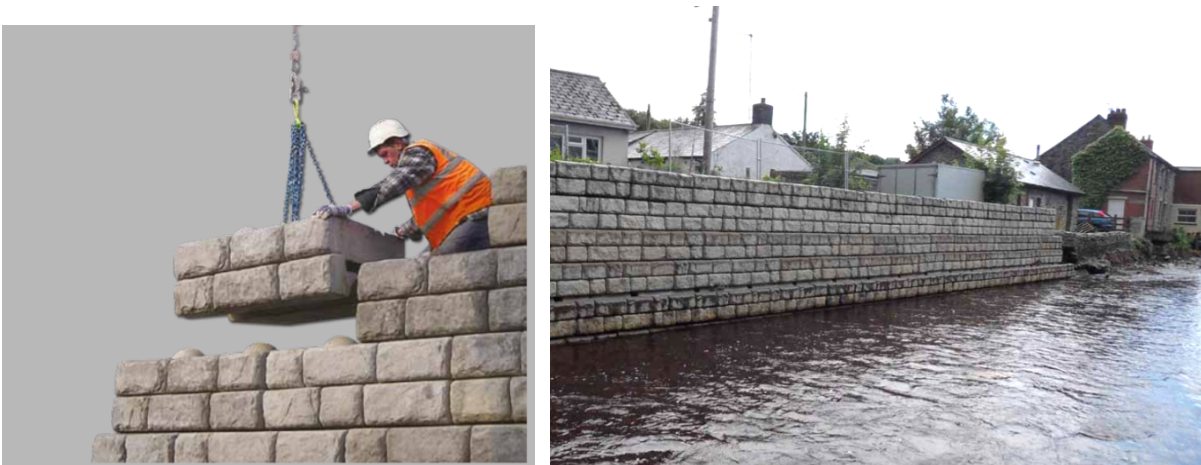
Figure 6.6: LEFT: Example of build-up interlocking modules. RIGHT: Example of application modules to retention wall. Retrieved from CPM (n.d.-c).
