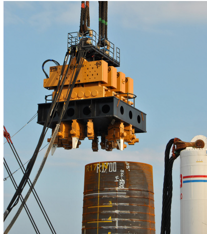
Figure 2.23: One of Cape-Holland its Vibro hammers for the installation of the Riffgat OWF in Germany Source: Cape-Holland
