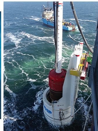
(b) Hydrohammer installing monopile through NMS Source: Energy-oil-gas.com
