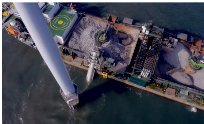
Figure 2.30: Scour protection installation with RSDU on the Seahorse Source: Tideway
