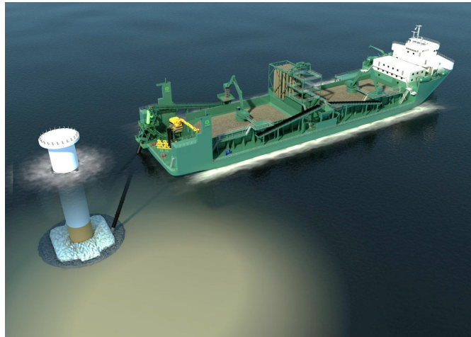
Figure 2.29: Scour protection installation with IFPS on Tideway Rollingstone Source: Tideway
