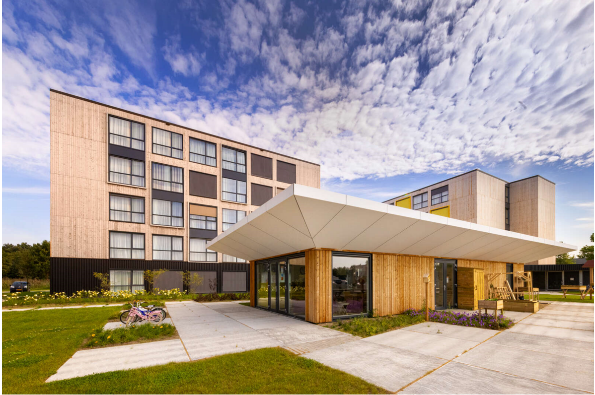
Figure 4.8: An example of a modular building developed by Daiwa Modular Europe. This project contains care apartments (Daiwa Modular Europe, 2023)
