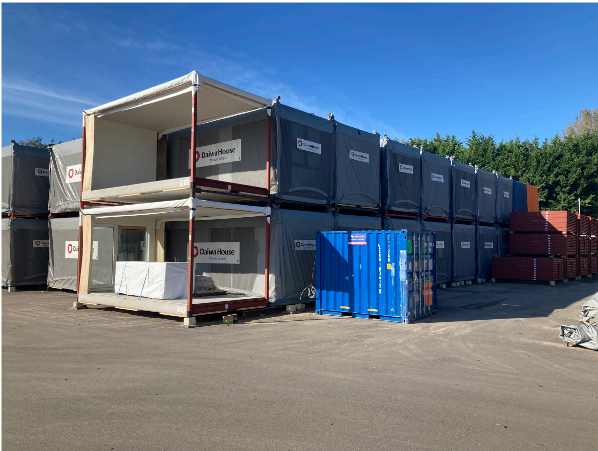
Figure 4.7: Once the volumetric units are manufactured they are stored on the site (Own work)
