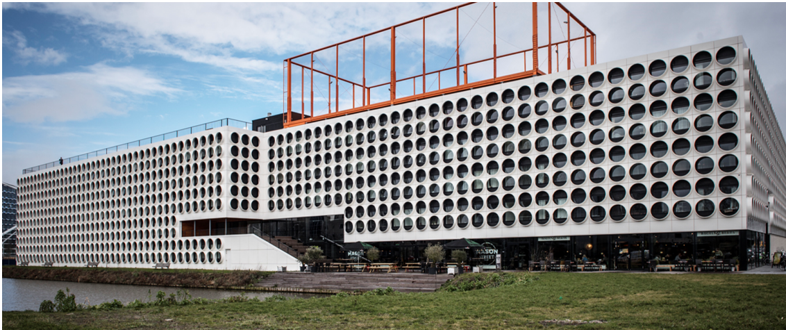
Figure 7.1: The Ravel residence, located in Amsterdam, needs to be relocated within 5 years
