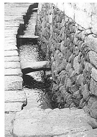
Fig. 5: Flowing water in ditches.
