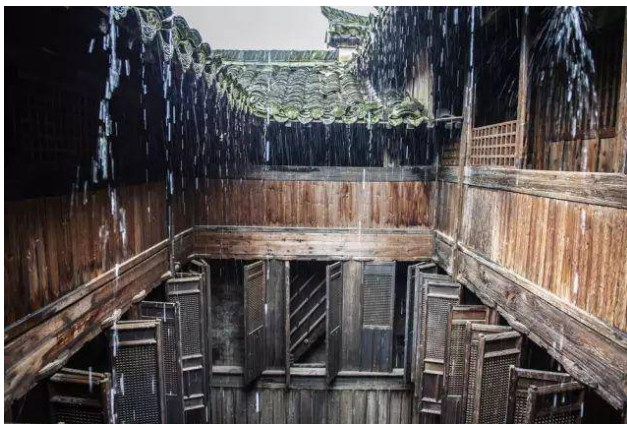
Fig. 6: The pitched roof and the rain curtain.
