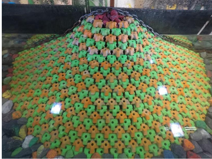
Figure D.61. Structure after 1.2 H_{m0} test run of Series 2.3 ( N_s = 2.83 ).
