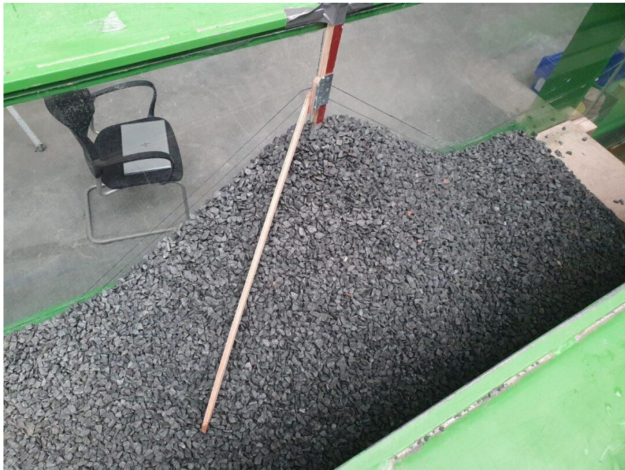
Figure 4.5. Tool to ensure a conical shape of the core applied in practice.
