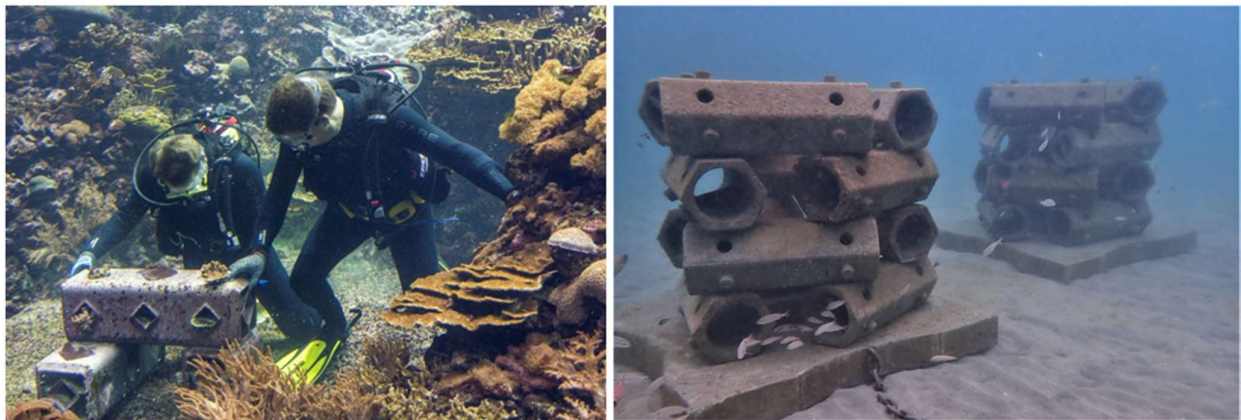
Figure 5.9: Different types of Artificial reef designs. On the left Reefy's design ( www.reefy.nl ). On the right Reefsystem's design (retrieved from www.reefsystems.org ).
