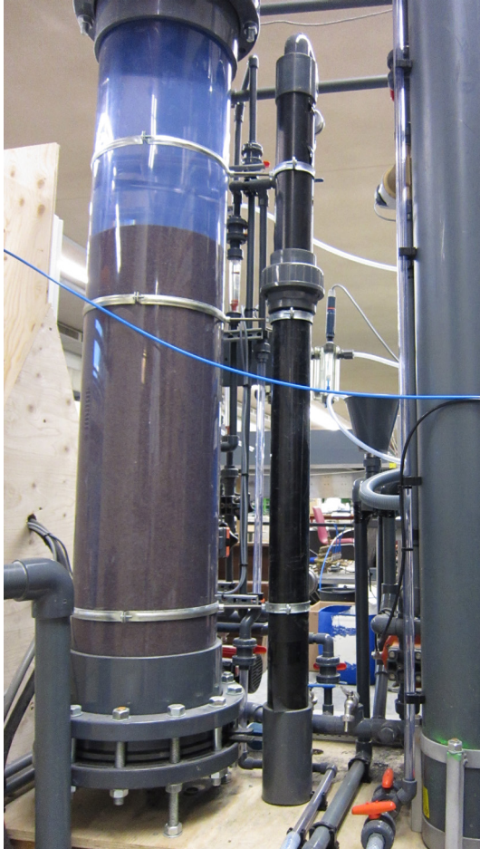
Figure 5: Biological activated carbon filtration as side-stream filtration
