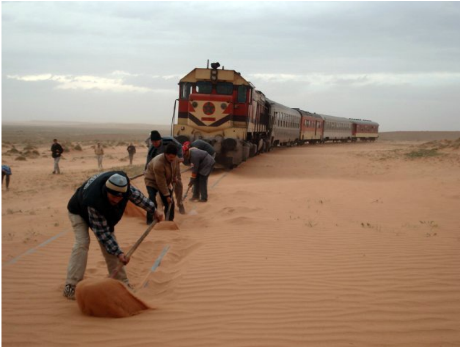
Fig. 28. Locals clearing up the Mediterranean-Niger Railway. Source from Oriental.ma.
