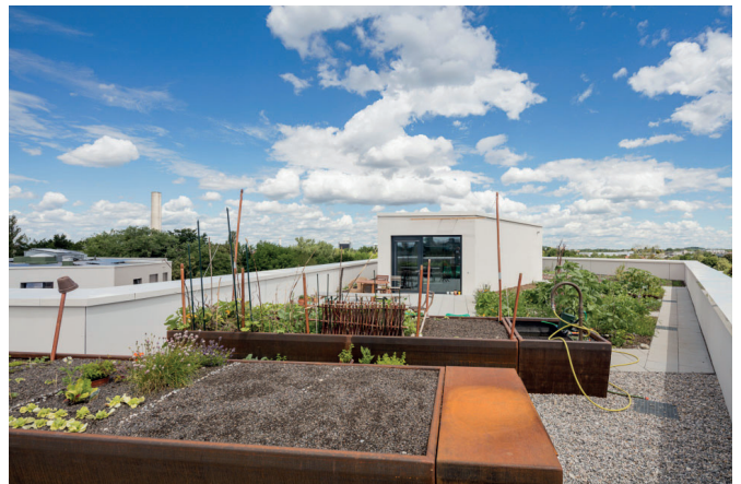
Figure 78: Shared roof garden (Archdaily, Gonzaléz)
