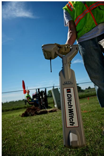
Figure 3.1: Walkover locating system in use (Underground Infrastructure Magazine [2012])
