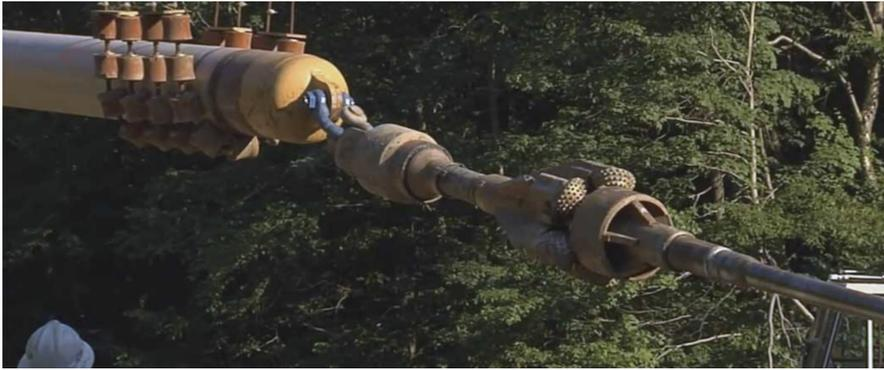
Figure 2.12: Reamer connected with a swivel to the product pipe (Kezdi [2020])
