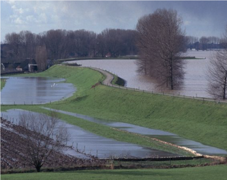
Figure 2.1: A long river levee (source: Rijkswaterstaat), from Schweckendiek (2014)
