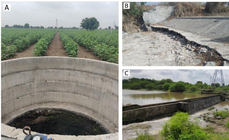
Figure 3.2: A) Open dugwell commonly used for irrigation in the Bhadar basin; B) and C) check dam in the area in dry and wet season, respectively (images taken from downstream side).
