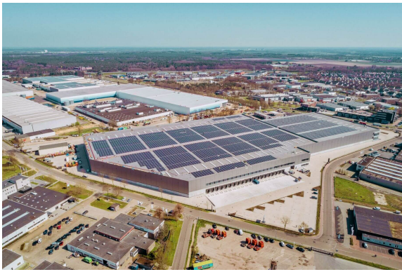
Figure 5.1: Logistical building similar to company X
