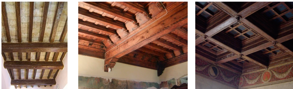
Figure 2.4: Different types of monumental timber floor structures (Left) Common timber-beam floor (Middle) Decorated and carved timber-beam floor (Right) Bi-directional timber-beam floor (Corradi et al., 2019)
