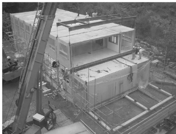
Figure 6: School in South Korea built using structural steel modules [3].
