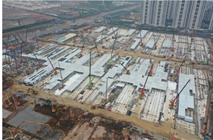
Figure 8: Leishenshan Field Hospital in Wuhan (China) built in 12 days [13]
