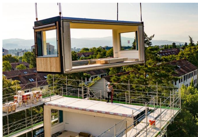
Figure 47: Corner supported Glulam module (Lehmann Group CH)
