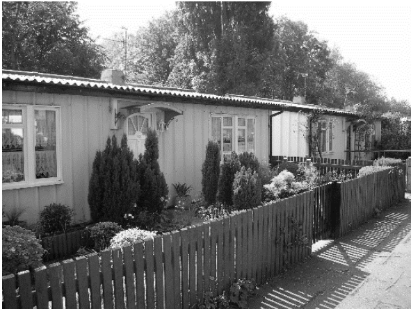
Figure 4: Phoenix system of prefabricated post-WWII housing in the UK. Steel frame and panelling [6]
