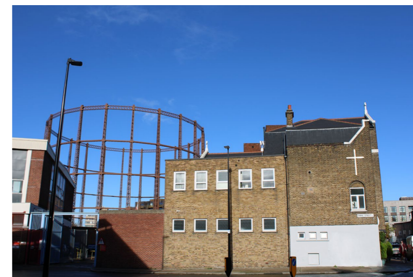
View from Hackney Road The lightweight structure of the Gasholder seen in the background gives a glimpse of the industrial heritage of the area while contrasting with heavy brick building in the foreground.
