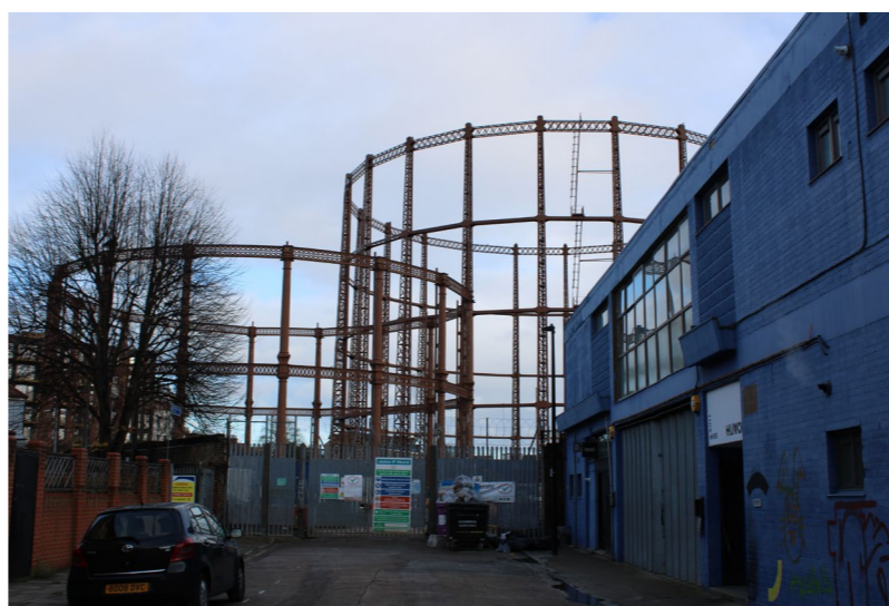
View from Marian Place Gasholder No. 2 and 5 seen from the main entrance of the gas storage station site
