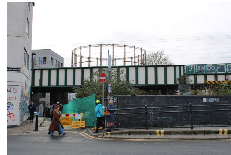
View from Cambridge Heath Road In combination with the rail bridges and roads, the gasholders form a complete image of the industrial legacy of the area
