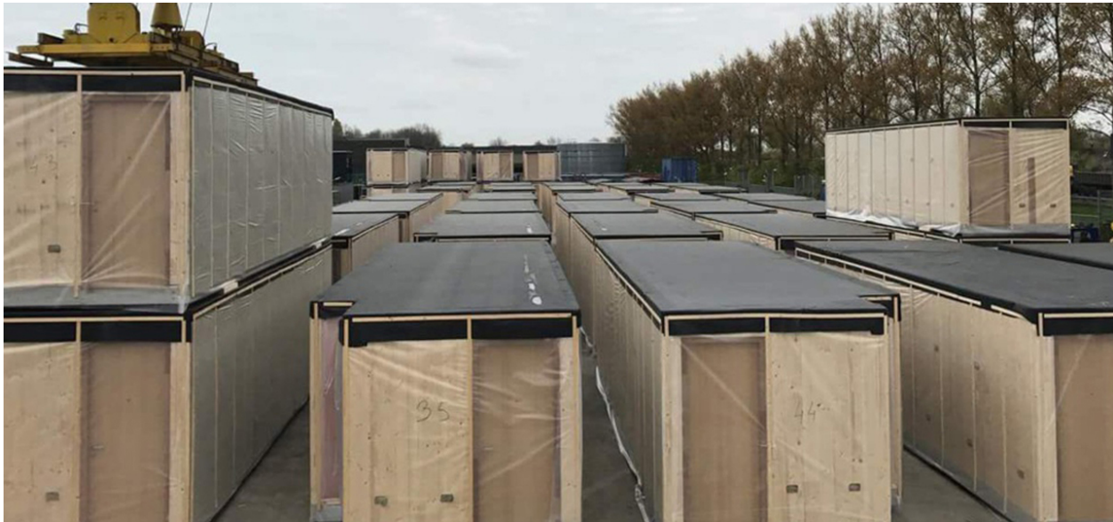
Figure 4.5: Modular hotel rooms (Hotel Jakarta, n.d.)
