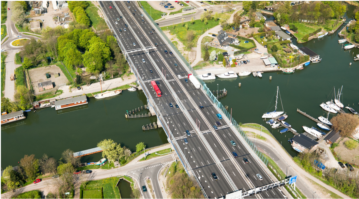
Figure 3.2: Vechtbrug in use in 2011 [15]
