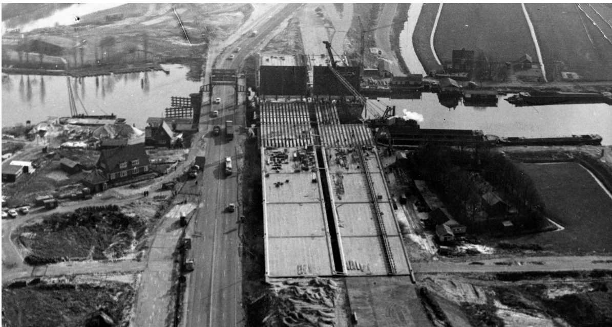
Figure 3.1: Vecht bridge under construction in 1965 [6]
