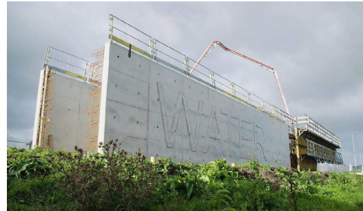
(b) Extinguishing water storage tank [6].
