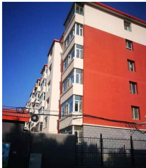
Figure 7. The residential building renovated in the case study (by the authors).
