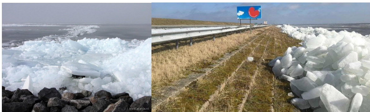
Figure 2. Photos of ice pile up on Afsluitdijk slopes
