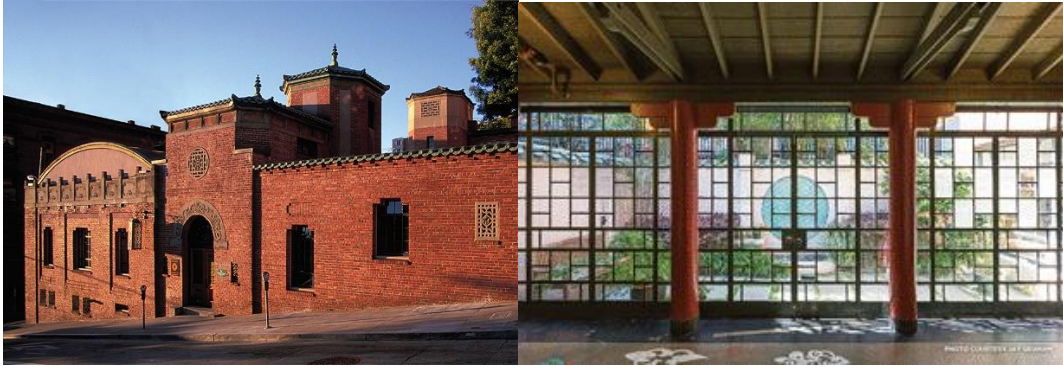
Figure 10: (Left) YWCA building, now the Chinese Historical Society of America building (About CHSA). Figure 11: (Right) Internal courtyard of YWCA building (Drueding).
