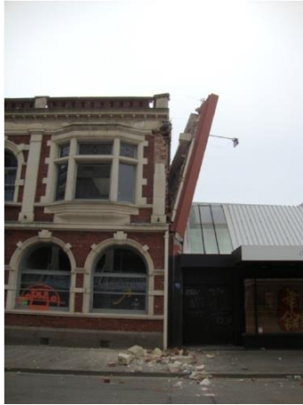
Figure 2.12 Typical failure patterns of an out-of-plane loaded wall subjected to face loads. [18]
