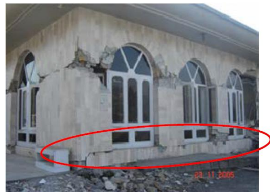
Figure 2.13 Typical failure modes of an in-plane loaded URM wall [20]
