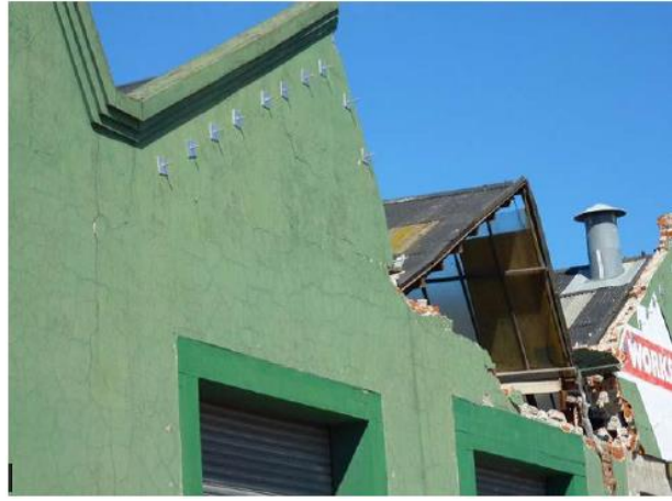
Figure 2.12 Typical failure patterns of an out-of-plane loaded wall subjected to face loads. [18]
