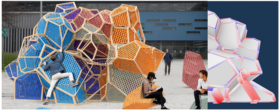
Fig. 2 Proposal for structure that can be partially dis- and reassembled with various functionalities (left) and structural performances (right)
