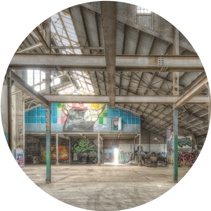
Exposed Steel Structures
