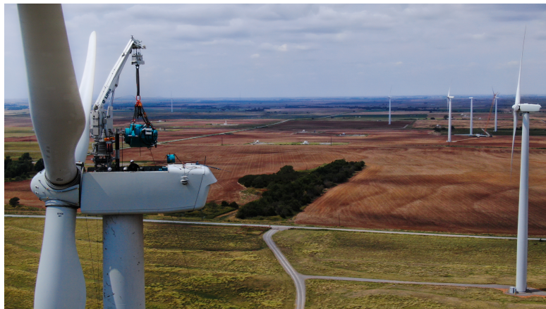
Figure 1.3: Gearbox repair/ replacement done by technicians using a self-hoisting crane (Enel, 2023)
