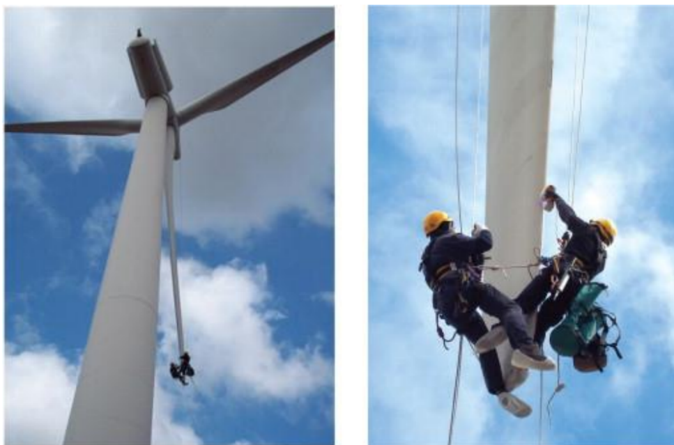
Figure 1.1: Technicians inspecting, cleaning and repairing the composite rotor blades.(Marsh, 2011)
