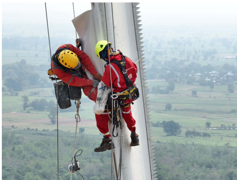
Figure 1.4: Blade repair done by technicians using rope (Vivablast, 2023)
