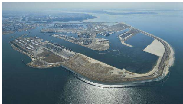
Figure 5.12: Aerial picture of Maasvlakte 2 in the Netherlands.
