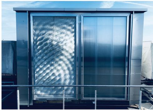
FIG. 16 Final Prototype of 3D Printed Future Façade
