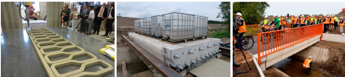
Figure 2: From left to right: printing of an element of the bridge, full scale test before final use, finished bridge. Reproduced from [5].
