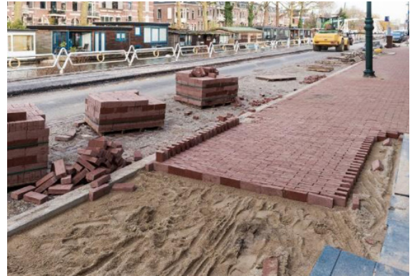
Figure 2.15. Brickstone replacement on pavements 9
