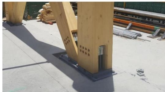
(b) Steel plates and dowel connection of diagonals [85].
