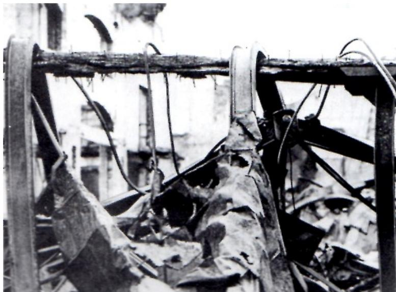
Figure A.5: Timber beam supporting melted steel beams after a fire in American factory
