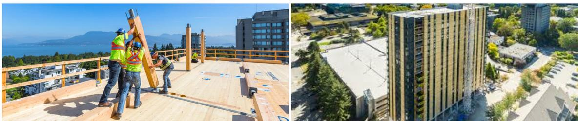
(a) Installation of glulam Columns [25].
