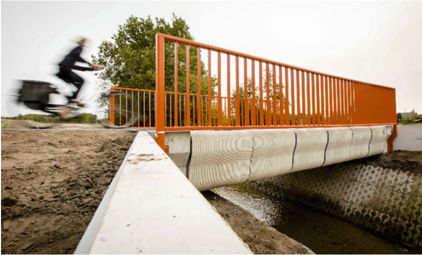
Fig. 2.2 Completed bridge at the opening. Photo Kuppens fotografie
