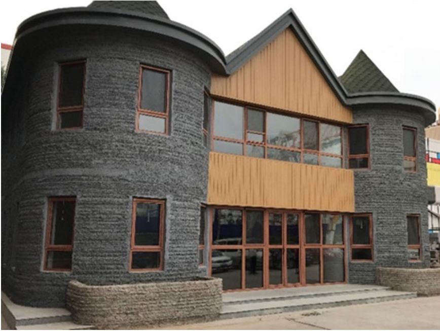
Fig. 2.22 The completed two-story villa
