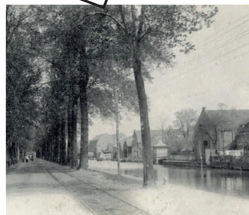
View on the Vaartsche Rijn, where the straight line of the canal is accentuated with a large tree line
