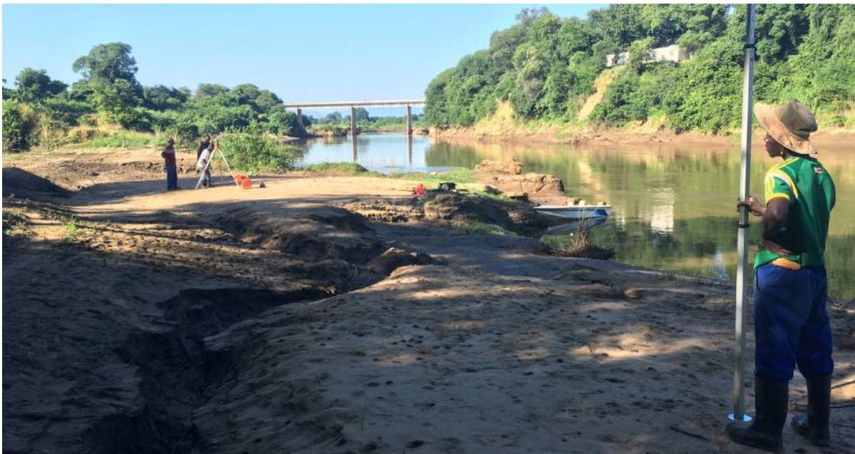
Figure 6: Determination of the three-dimensional coordinates of a GCP (CD underneath the pole) on a floodplain of the Manyame river downstream of the Mushumbi bridge.
