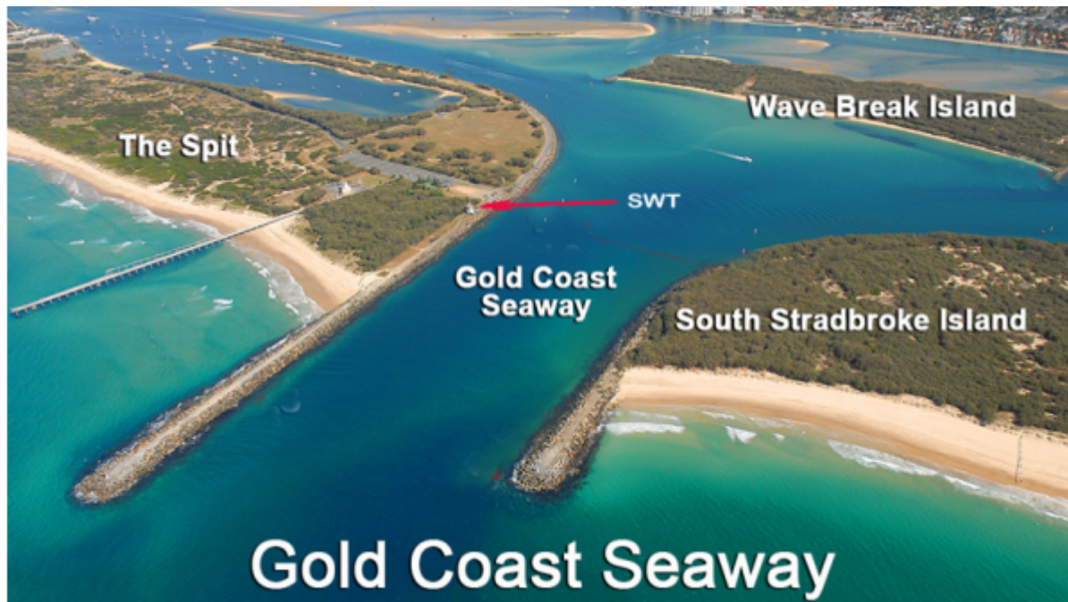
Figure C.5: Overview of the sand bypass system in Nerang River (Soares, 2017)
