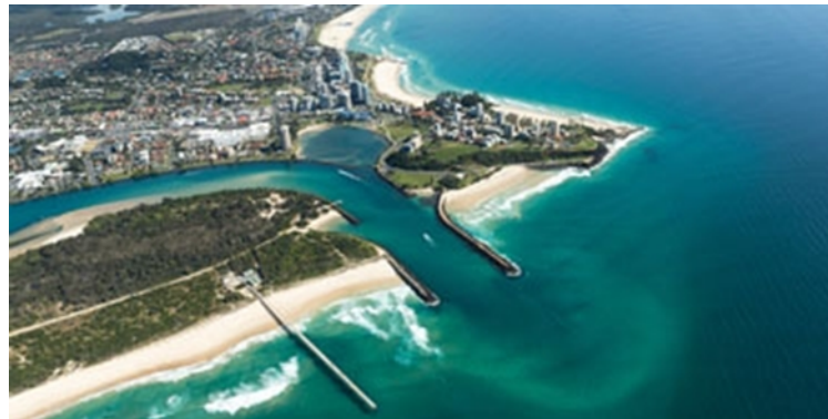
Figure 1.2: Fixed sediment-bypassing jetty at Tweed River Entrance Project (Australia) (Government, 2022)
